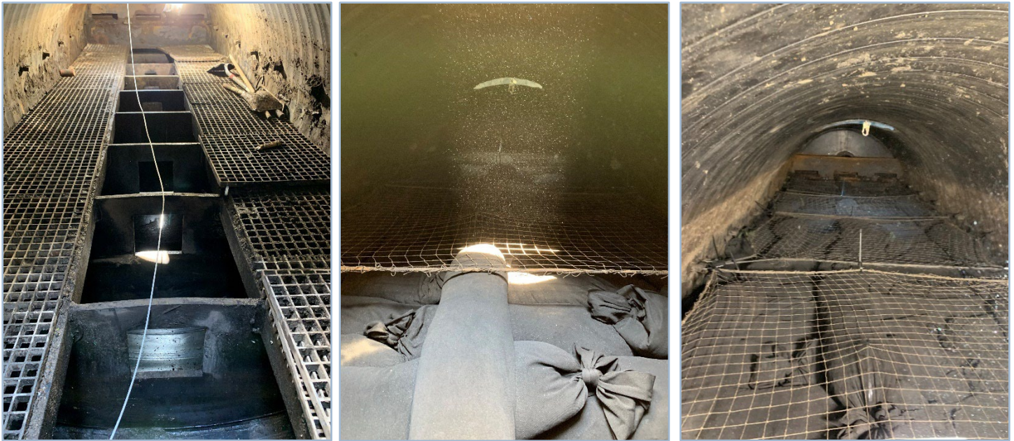
Picture 4.1, 4.2, and 4.3: Inside view of the Aqua-Filter filtration chamber; Biochar being placed in the filtration chamber; Biochar secured in the filtration chamber.
