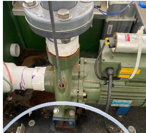
Steel rod to free impeller
