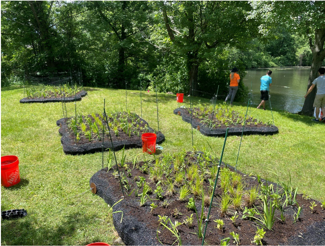
Photo 2.2: New FWIs planted and ready for installation
