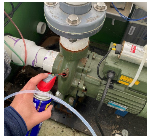
Spray lubricant into pump housing
