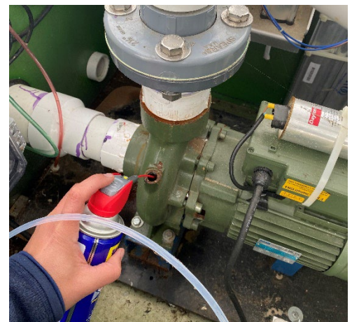
Spray lubricant into pump housing
