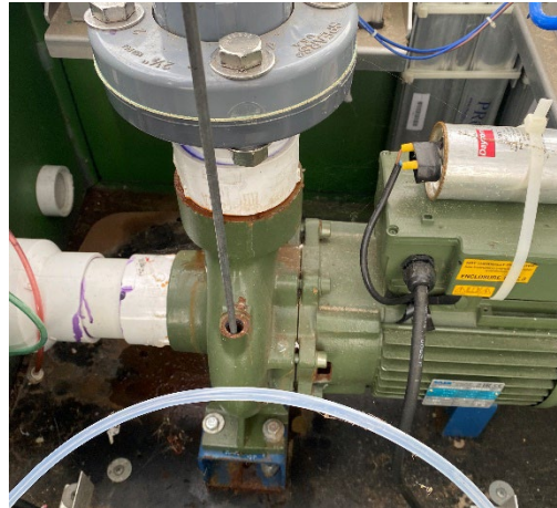
Steel rod to free impeller
