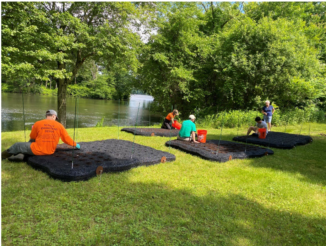
Photo 2.1: Preparing the new FWIs with a soil and peat moss mixture
