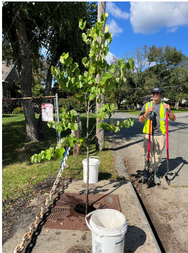
Photo 4.2: Completed tree planting in a Filterra unit in October 2023
