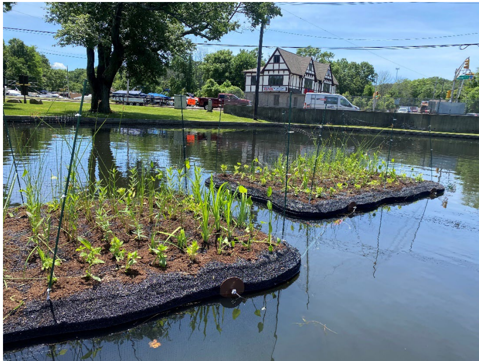
Photo 2.2: Finished FWIs installed in Landing Channel in 2022
