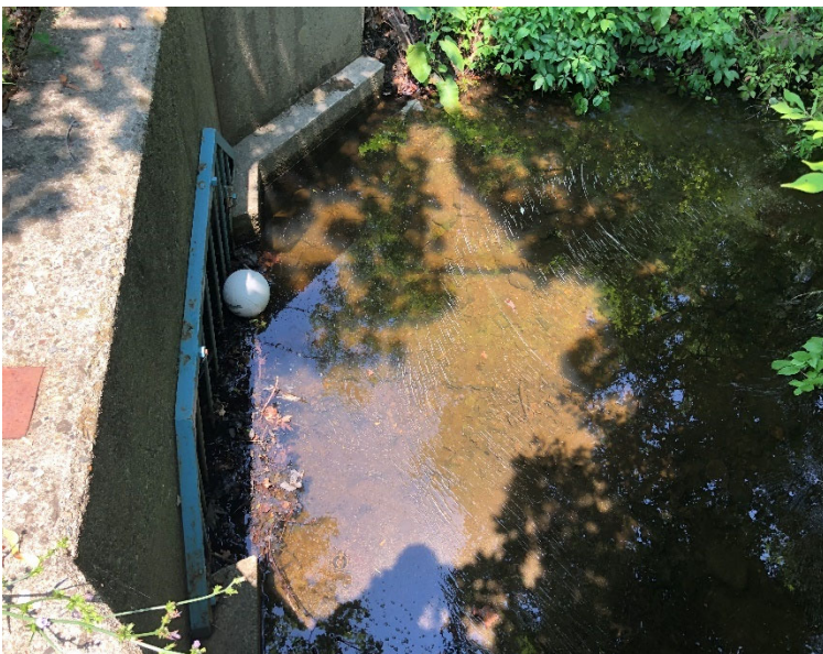
Photos 2.6 – 2.7: Culvert at the S-3 stream in July (left) and August (right) with significant sediment accumulation
