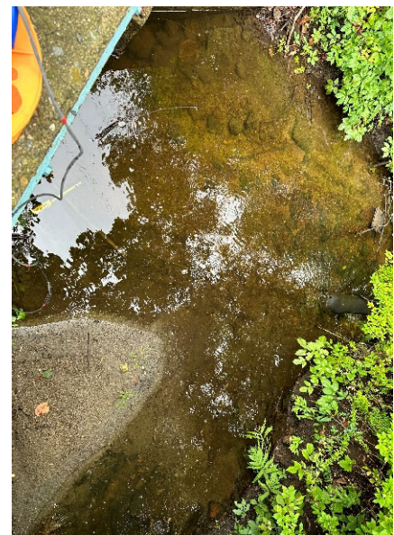
Photos 2.6 – 2.7: Culvert at the S-3 stream in July (left) and August (right) with significant sediment accumulation
