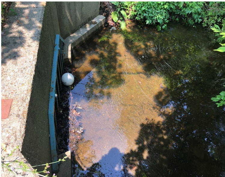
Photos 4.3 – 4.4: Culvert at the S-3 stream in July (left) and August (right) with significant sediment accumulation
