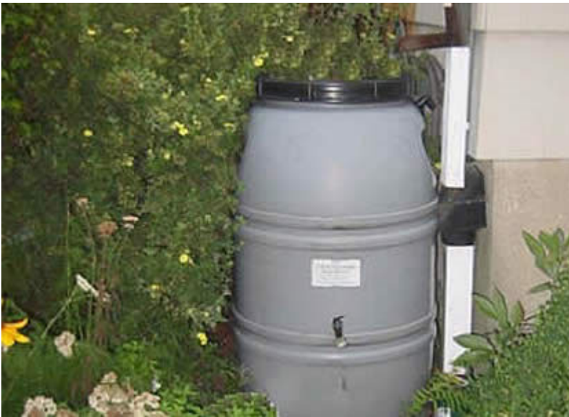
Photos 4.14 – 4.15: Rain barrel (left) and cistern (right), Sources: CT DEEP (left) and USEPA (right)
