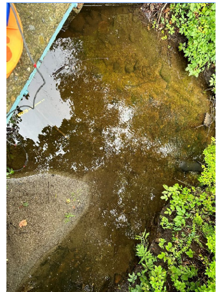
Photos 4.3 – 4.4: Culvert at the S-3 stream in July (left) and August (right) with significant sediment accumulation
